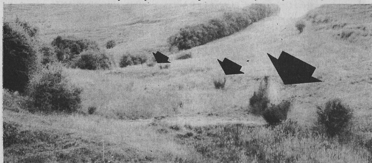
Simultaneous explosions in a difficult stretch of terrain – difficult because of a swamp area. The arrows show the blow-ut of sand where each piece of 'jelly' was planted.
