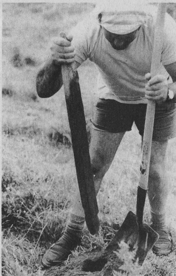
Small charges of Gelignite are placed and wired then the holes are filled with sand & rammed.
