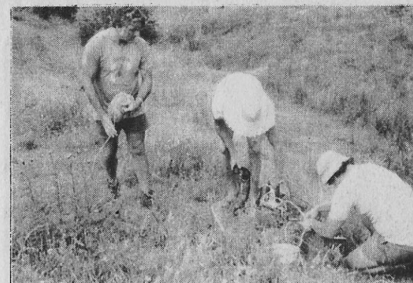
The final stages of wiring and preparing to blow the charges. Above right we can see one member of the team in phone contact with the control base. It is from this control base that the charges are actually fired, after that is, a warning blast of vehicle horns has been sounded.
