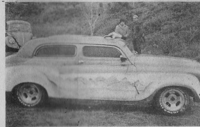
A wildy customised 1954 Hillman 80. The roof has been 'chopped' nearly five inches.
