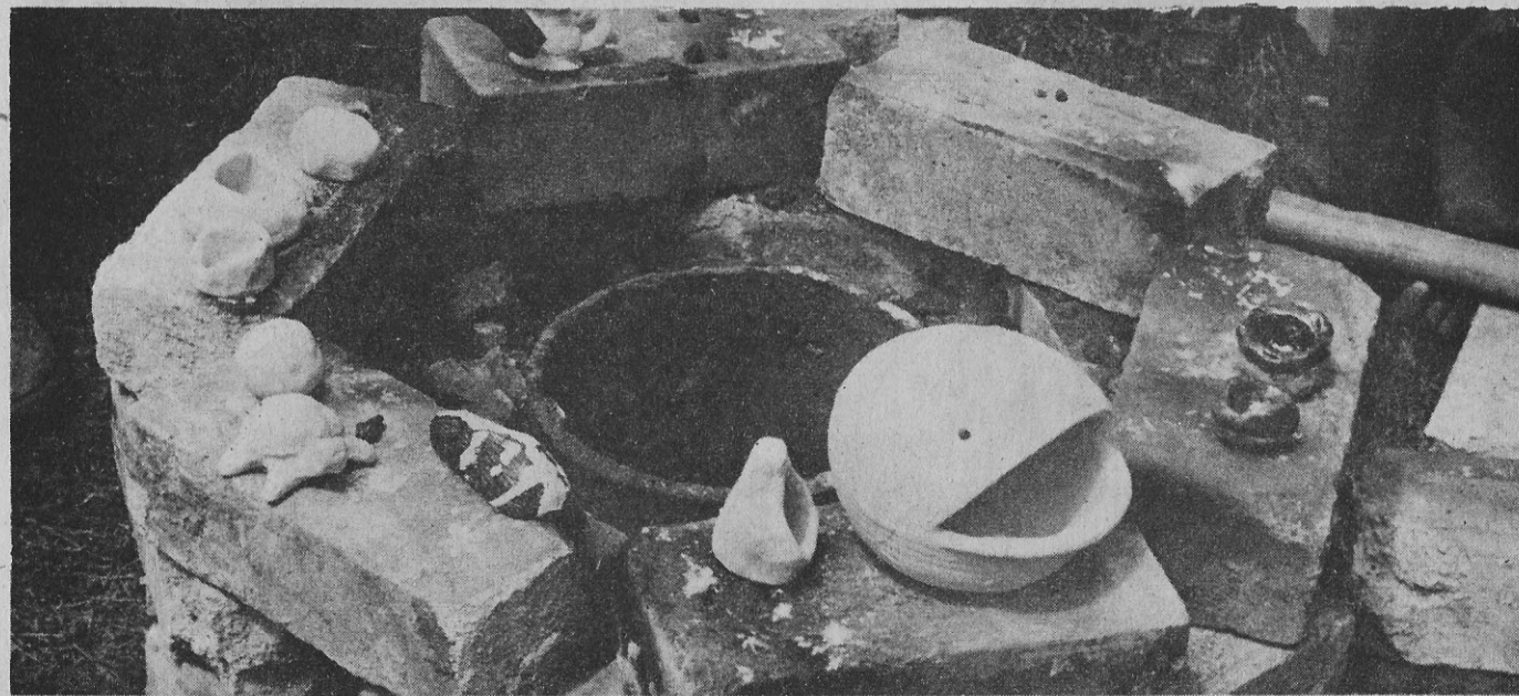
It is in this pot that the glaze is melted onto the clay of the pottery.
