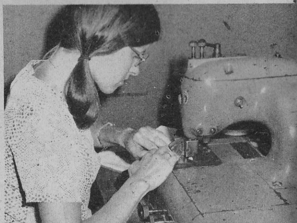
Janice Kendall on the skiving machine which makes a groove around all the edges to make them neat when folded
