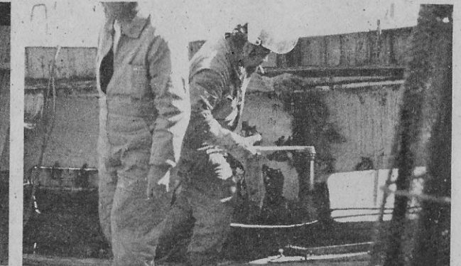
Welding in progress on the hull of the boat
