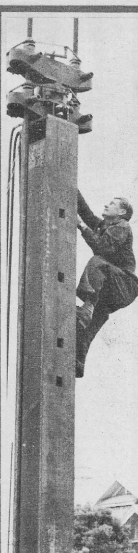
Lift Slab engineer Mr N. Blackburn of Sydney goes up the girder, to see to one of the lifting jacks.
