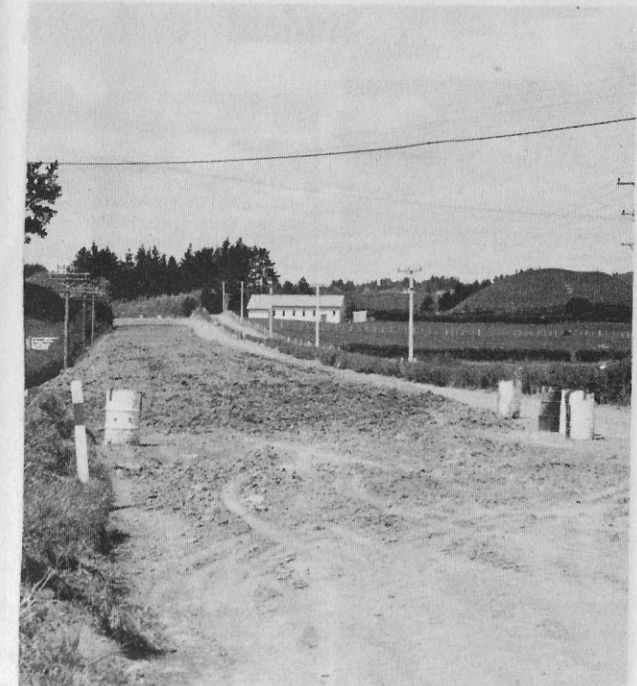
Going north off the end of the Mangorei straight a new cutting will keep the road straight, instead of the present number of dangerous curves that formed that part of the road.
