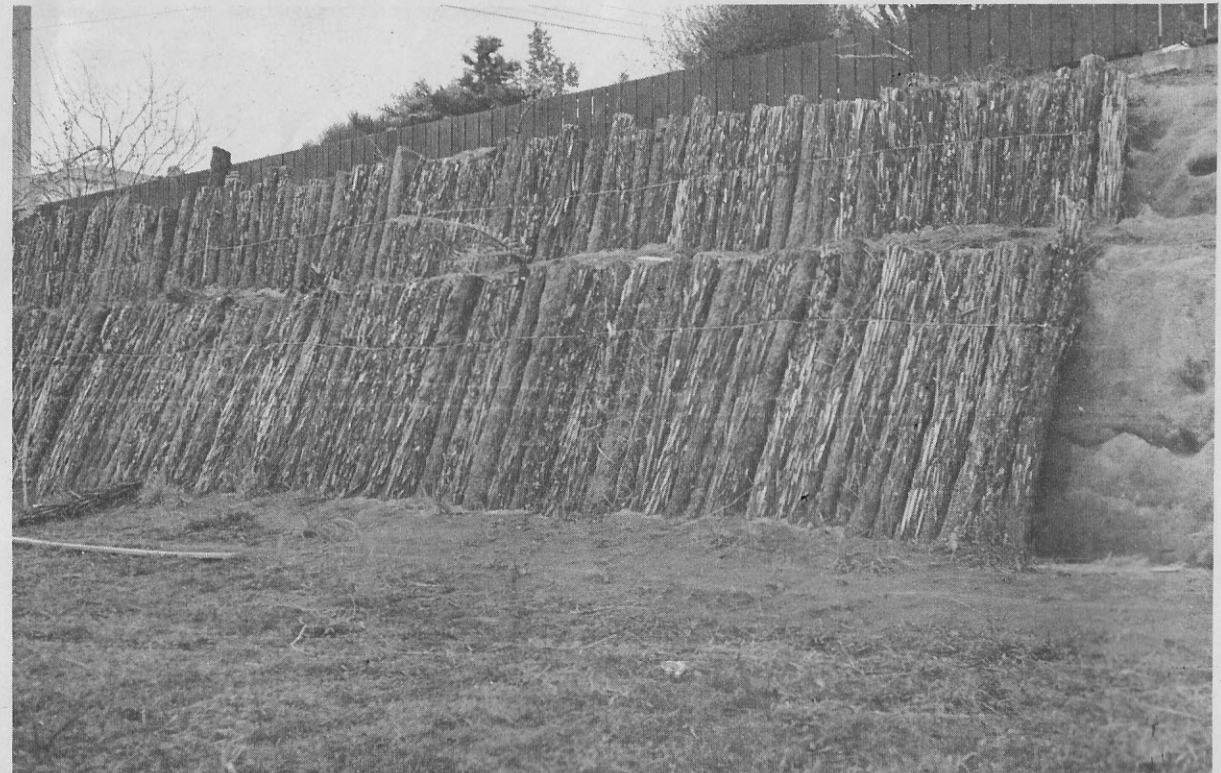
So far, some levelling of the section has been achieved and a retaining wall built
