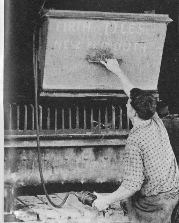
Basil Martin at work on the hydraulic cement conveyor prior to mixing
