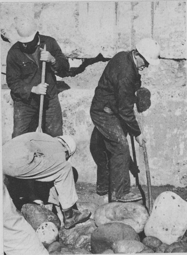
Above, left: There's a lot of crowbar work, placing the smaller boulders in position. Something like 2,500 tons of boulders a day are being put in place in this extension work.
