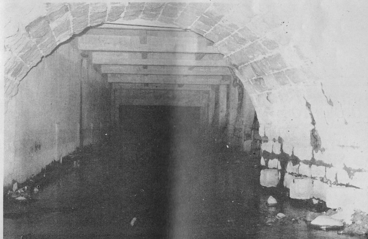
And this was the under-side of the old Huatoki bridge
