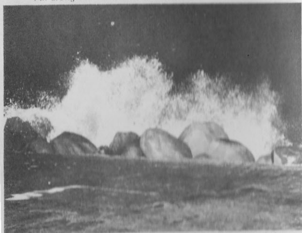
At the Port, waves smashed against the outer wall of the breakwater
