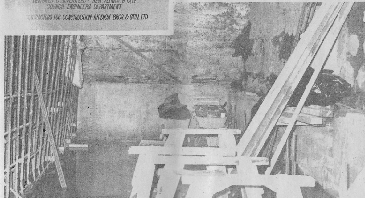
New construction work is pictured here
