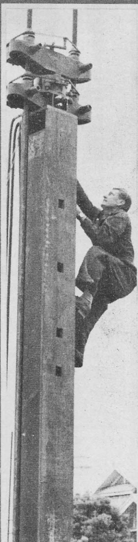
Lift Slab engineer Mr N. Blackburn of Sydney goes up the girder, to see to one of the lifting jacks.
